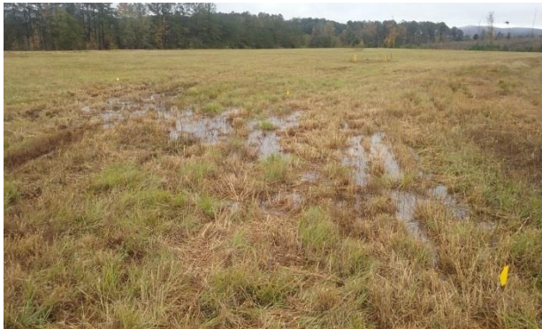
LF3_11.2.2015-002: Several areas were observed to be holding water after the rainfall event. The areas holding water were near the block and gravel inlets. This view is located in the west-central portion of the landfill looking to the south.
